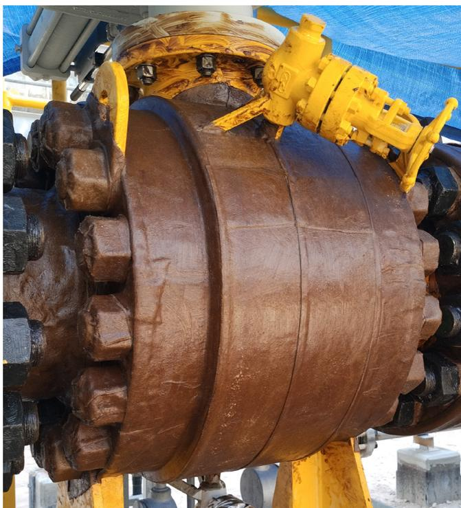
A 24" pipe valve was coated with the Temcoat™ 3000 primer and Wax-Tape® HT-3000 wrap system. The conformability of the wrap meant that it could be applied without a mastic, making the application process fast and enabling a rapid inspection.
