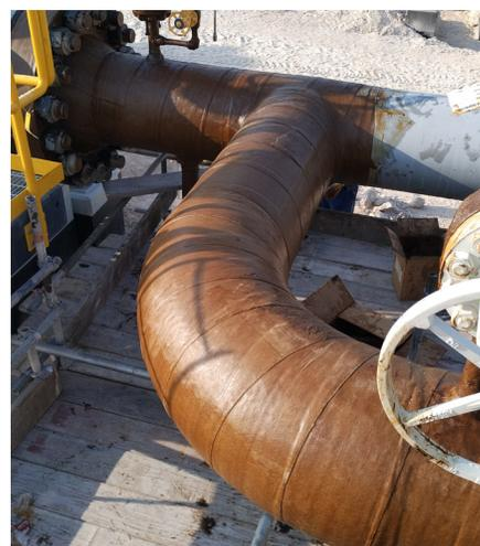
In tight quarters, the advantage of the Trenton Wax-Tape® wrap system over other solutions is the ease of surface preparation and application as compared to an abrasive blasting or a bulky wrapping machine.
